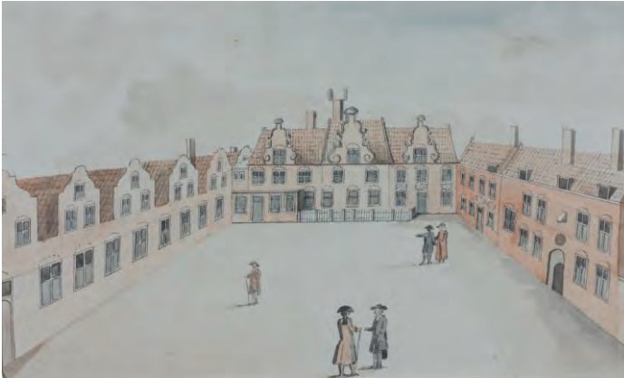
Figure 33b. The inner courtyard of the State College, viewed from the north. Watercolour drawing by Jacob Timmermans, 1788. In the background, the southern building is visible. It consisted of a lecture hall, probably with a small reference library, a kitchen, and a dining room. The director's residence on the left is inaccurately depicted. More realistic depictions appear in Blaeu's city map of Leiden (1649; Fig. 31d) and in the 3D model above. Source: Erfgoed Leiden en Omstreken (PV_PV16304). Courtesy of Erfgoed Leiden en Omstreken / Leiden Regional Archives.
